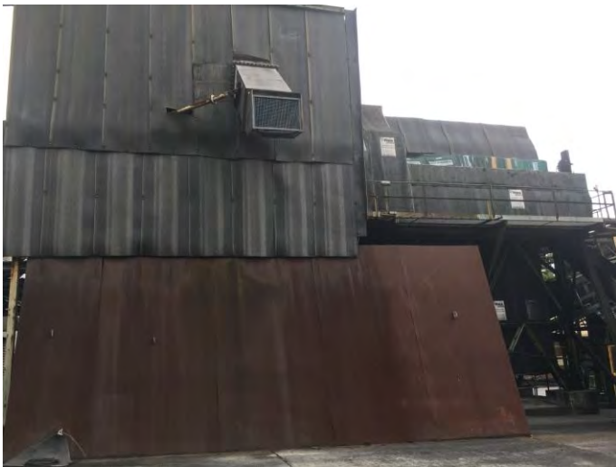
Plate 4.7 Noise mitigation cladding on CHPP
